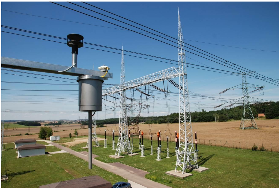
Figure 20: Installation of the PMS system on a high voltage substation.
