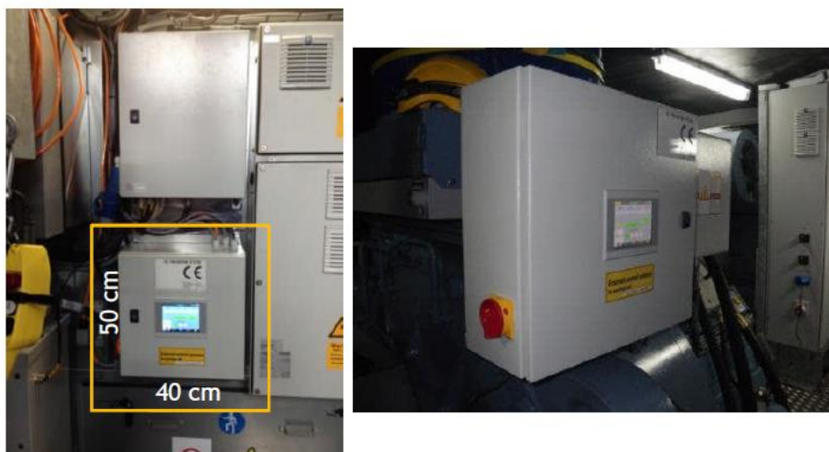
Figure 18: Cabinet of the IPMS system inside the nacelle of a wind turbine.
