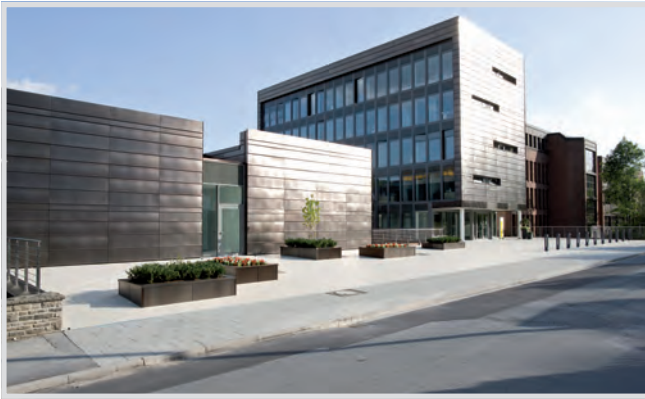
Fig. 5: The Training Centre of the KRAFTWERKSSCHULE E.V./ PowerTech Training Centre Association in Essen-Kupferdreh with the new building at the «Deilbachtal Energie Campus».
