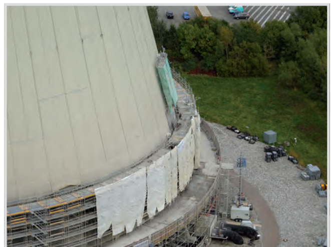
Fig. 8: Cooling tower of the thermal power plant Rostock under revision, detail, KNG.
