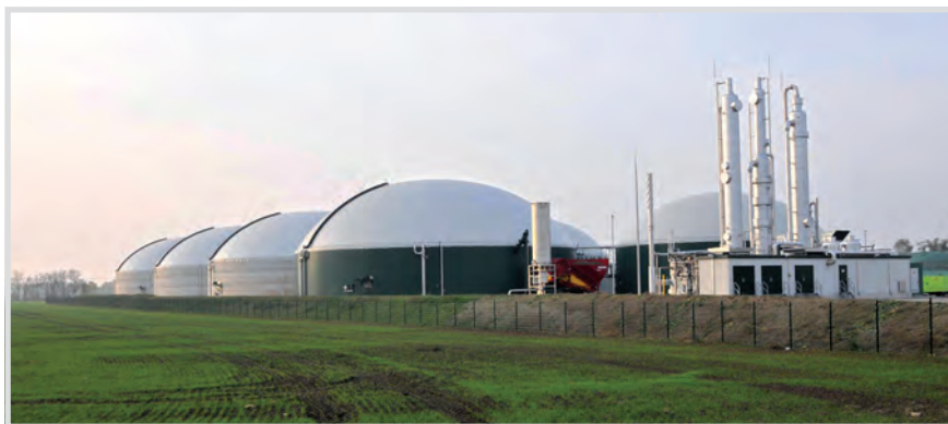
Fig. 14: Barby Biomethane Plant. Source: MVV
