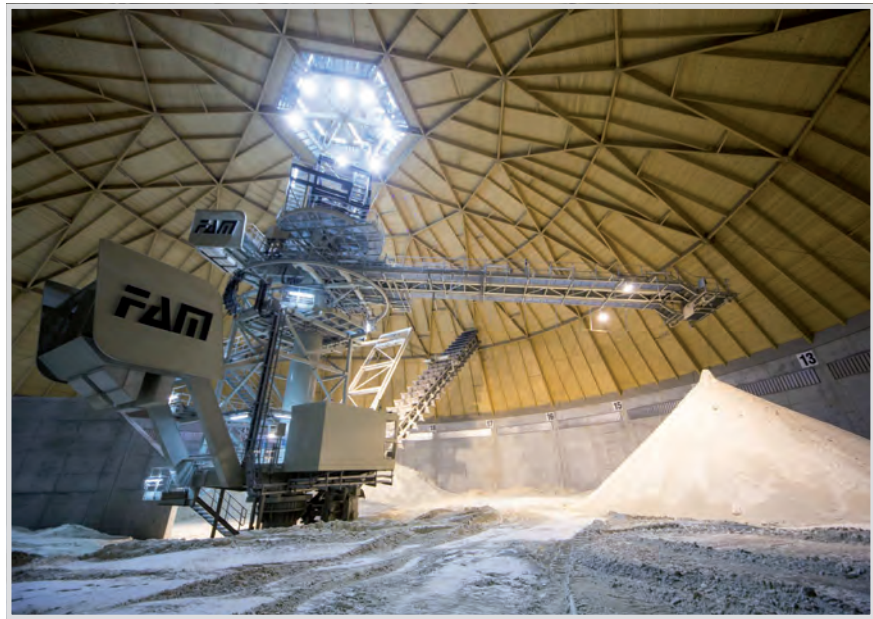
Fig. 5: Gypsum store at the Moorburg combined heating and power plant.
