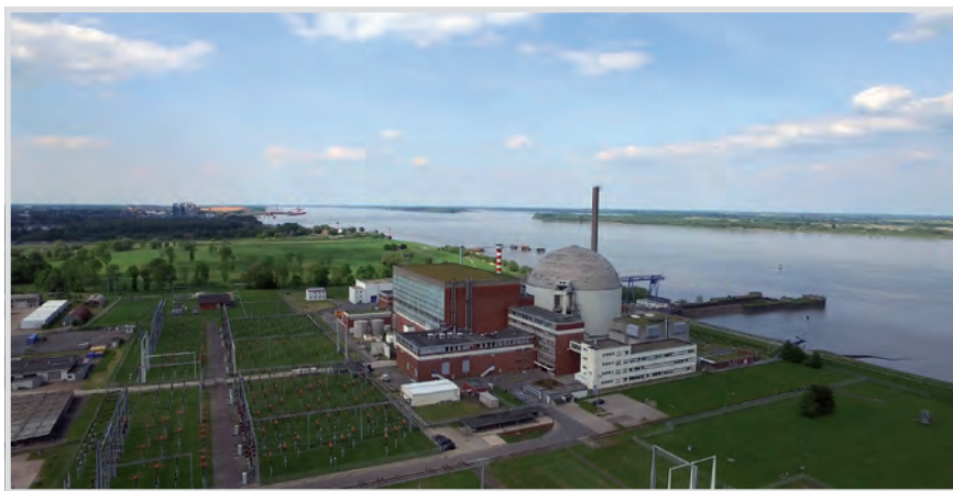
Fig. 8: Nuclear power plants in decommissioning, NPP Stade. (Photo: PreussenElektra).
