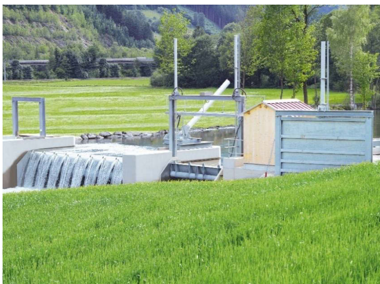
WKW Pollinger (Styria): Control for hydropower plant and cloud integration
