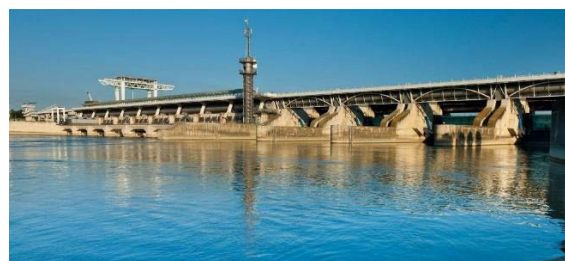
Freudenau hydropower plant on the Danube River (Vienna).
