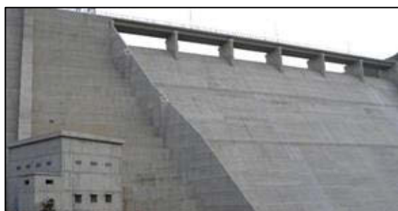
Barrage Ouljet Es Soltane, Maroc, 2017 (under construction at that time); © Bettina Geisseler.
