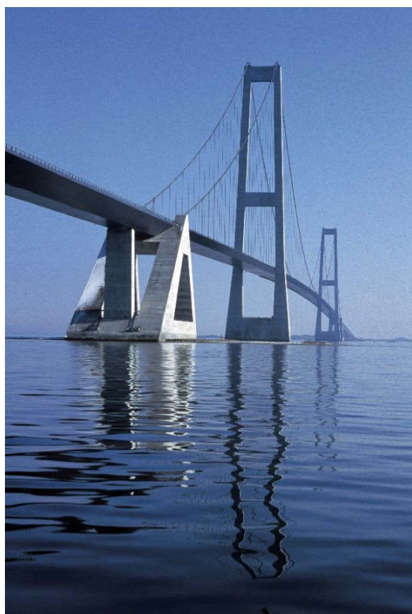
Storebælt Bridge, Denmark; © Sund & Bælt Holding A/S.
