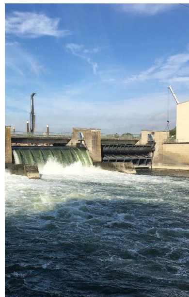
Delft-FEWS supports the operation of Run-of-River Power Plants.
