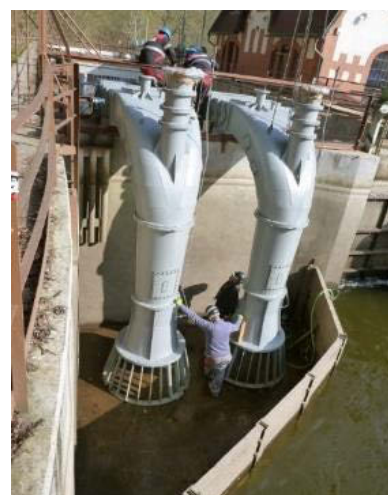
Installation of siphon low head turbine.
