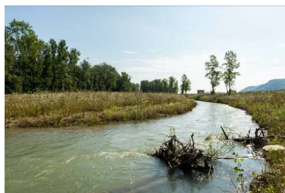
Fish bypass at the hydropower plant Greifenstein.
