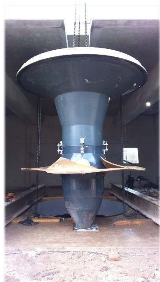
Vertical Kaplan Runner Ø 3,150 mm.
