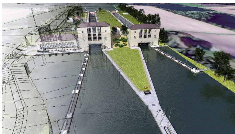
The Wedtlenstedt lock was built in 1939 and needs to be modernized and expanded. Our 3D model of the existing lock and the environment, generated from terrestrial photographs and videos, was used for early stakeholder engagement and communications.
