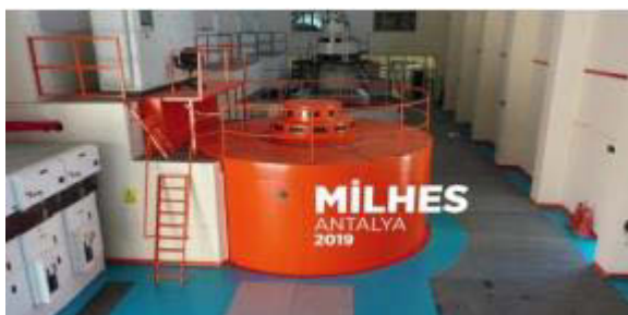
First national HEPP turbine and generator design, increasing the power output from 8.8 MW to 9.5 MW.
