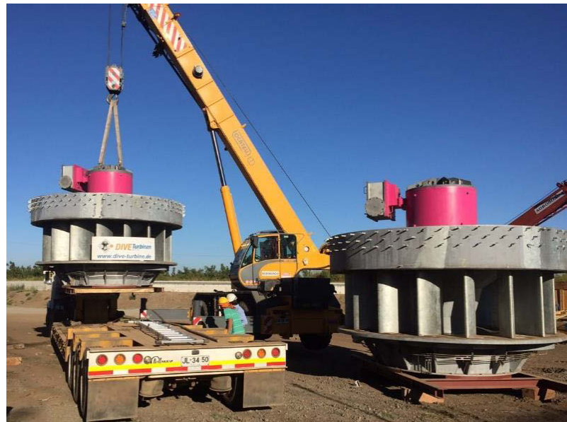
DIVE-Turbines in Chile: the turbines are fully assembled in factory. The tolerances to the civil works on site are very big.
