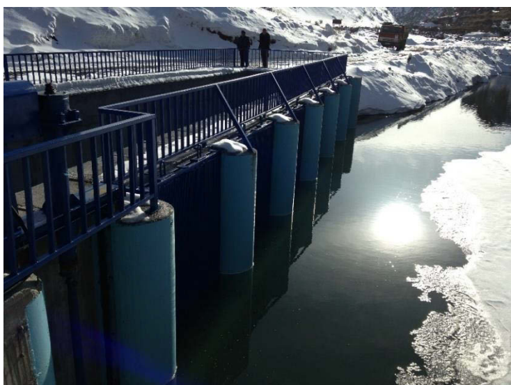
HPP Vardenik (Armenia): Control for hydropower plant and cloud integration
