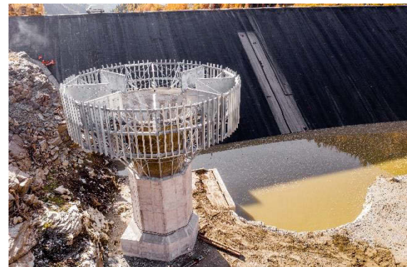
Restoration of the inlet guiding cone at Wurtenspeicher, Austria.
