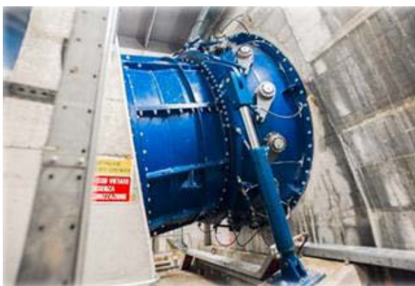
Wicket Gate mechanism for the same Turbine Runner Ø 2,800 mm 2,000 kW.
