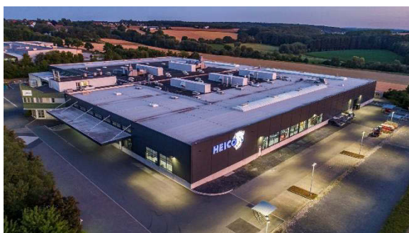
HEICO Group production site in Ense, North Rhine-Westphalia.
