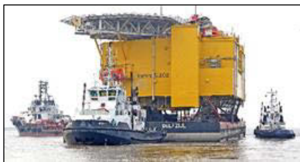
Converter Station offshore windfarm Meerwind Süd/Ost; © Alstom Grid (nowadays: GE Grid Solutions).
