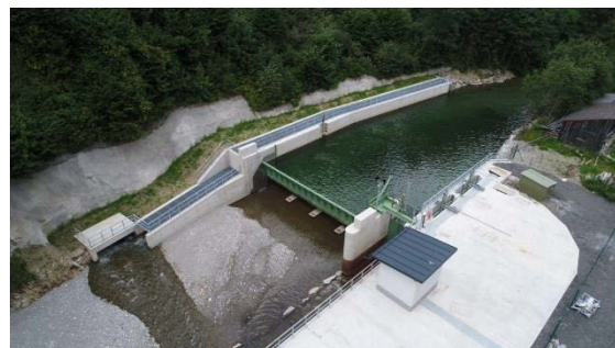
Intake with fish pass, hpp Kremsbrücke, Austria.
