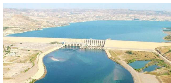
Birecik hydropower plant on the Euphrat River (Turkey).
